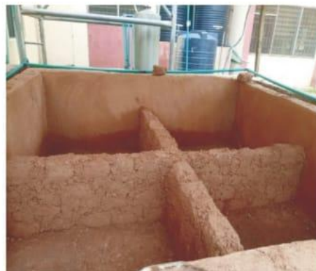
Figure 2b: Internal clay-based partitions of a typical ZECC
